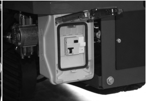
Fig. 82 Main electric switch
